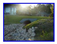
Phase II: <u>BMP Implementation</u>. The inflows leading to the Lake and the constructed sumps were reconstructed with the lime rock; a long unpaved access road to the dam on Lake Blue Heron was paved with granitic gravel to decrease erosion and dust. Berms and swales were built along the sides of the road to stop erosion; an educational outreach program was implemented to
