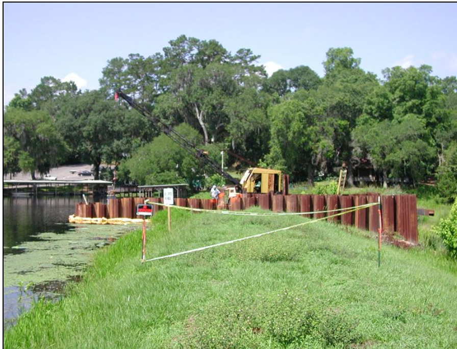
Figure 5.2.13: The northern dam on the sinkhole at lake Miccosukee failed. The old control structure rusted through and was replaced. The GFC repaired it. Lake water levels are normal (photo by Michael Hill, July 2004)
