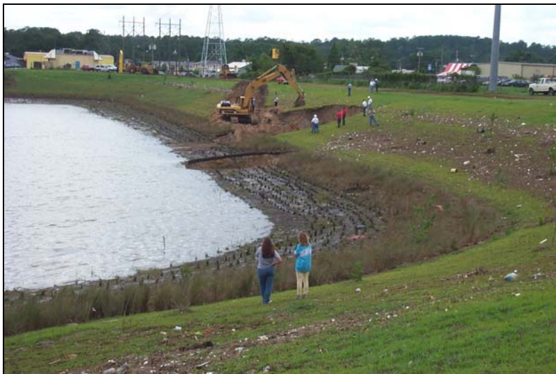
Figure 5.3.2A.5: Sinkholes in Elberta Crate Pond, 2002, when the contaminated soils were removed the resulting pond was developed over 30 sinkholes. These numerous sinks were filled with grout. Lime rock pinnacles weakened the clay liner. Similar conditions exist beneath the Civic Center and the Seminole Stadium. This implies caverns.
