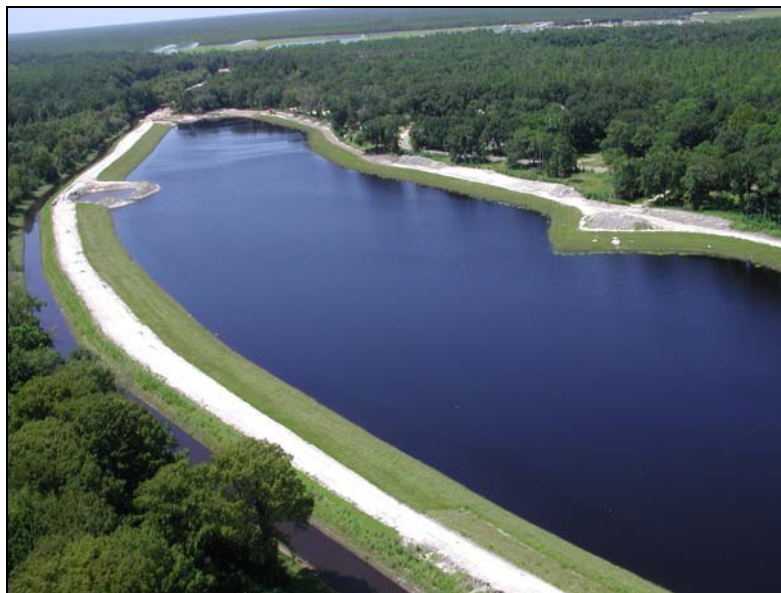
Figure 5.3.2A.7: The cypress trees in Lake Henrietta were cut down and it was modified into a stormwater facility. A large sinkhole that opened during construction is visible to the upper left
